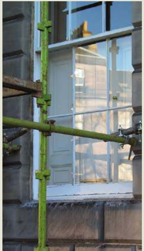
Scaffolding can be hazardous to old glazing
