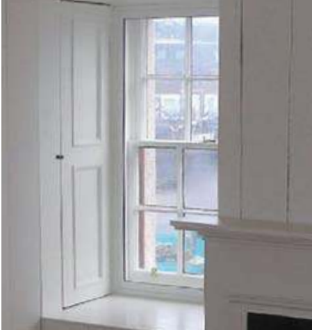
Secondary glazing can be effective and unobtrusive
