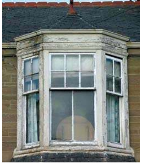
Deteriorating paint leaves timber vulnerable to decay
