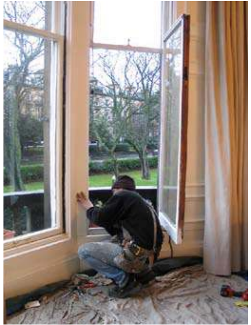
'Simplex' hinging system in operation
