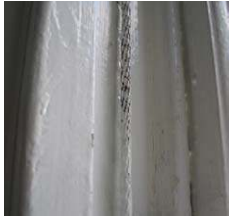
Paint-covered sash cords will make the window more difficult to open and close
